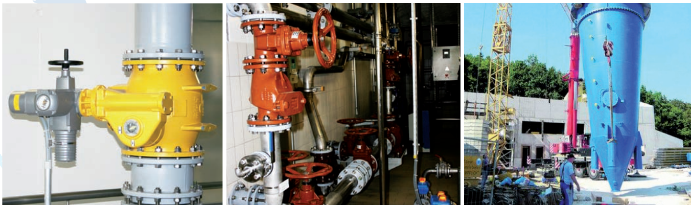
In September 2008, construction work began on the central „Sallmannsberg“ pumping station in the district of Blindheim. Following a two-year construction period, the highly modern water softening plant was started up in September 2010.
